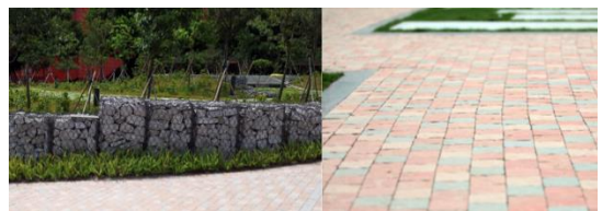
Gambar 21: Gabion wall and eco paver (Sumber: CIC-ZCP (Construction Industry Council & Zero Carbon Park, 2022)
